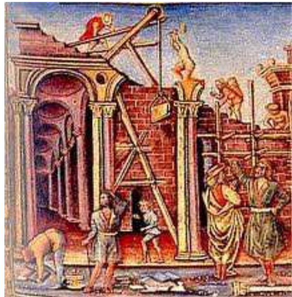
Operative masons at work.
